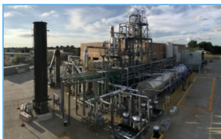
Alterra Energy's industrial - scale waste plastics liquefaction unit in Akron, Ohio. Photo: Alterra Energy
